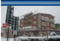
HOTEL ** Dosdè Motel GROSIO Via Milano, 105 Tel. (+39) 0342 847.380 www.grosio.com
